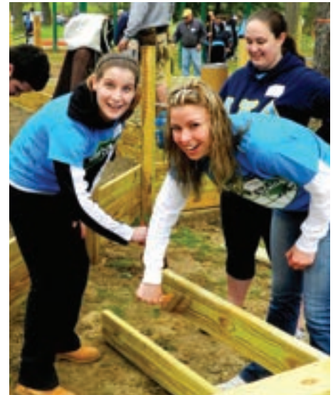
Above: Thiel students stain lumber for the project. Below: A portion of the volunteer army who helped build the Riverside Park playground. Inset: The finished playground.
